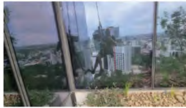
Australian customer performing exterior facade maintenance on high-rise buildings
