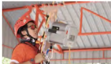
Maintenance and repair of wind turbines
